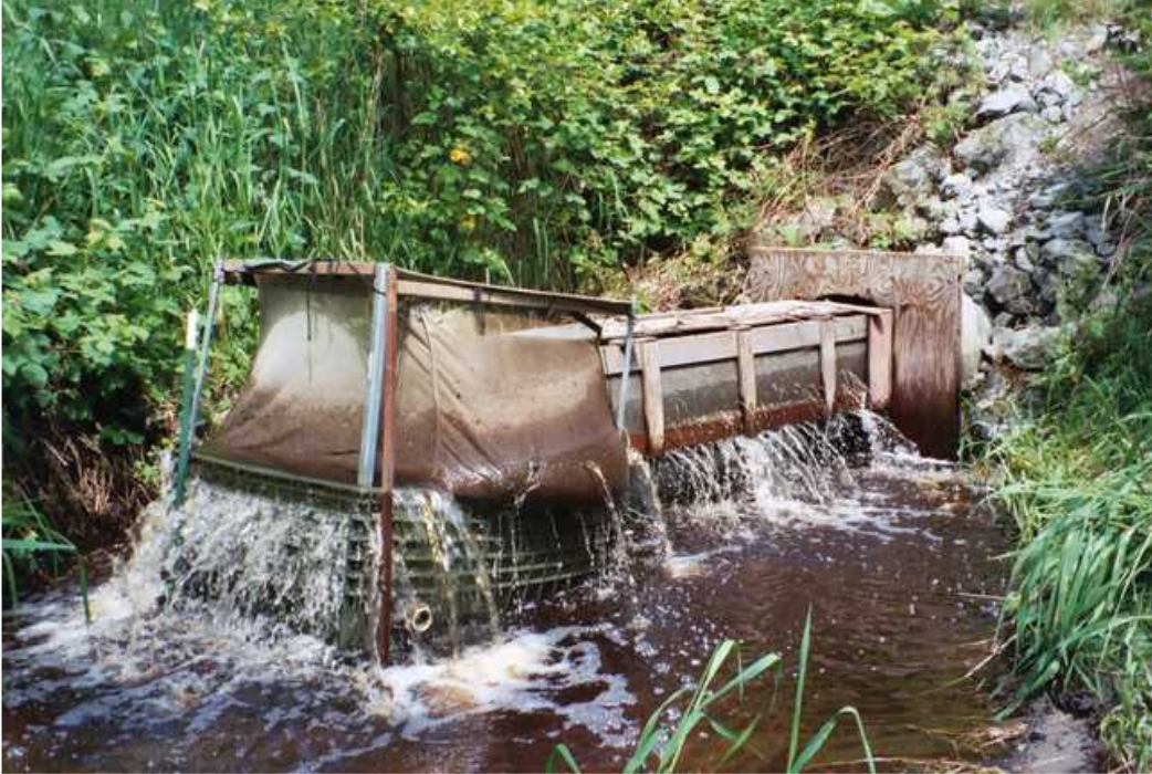
Figure 8. Whidbey Watershed Stewards smolt trap installed at the outlet of the French Rd. culvert on lower Maxwelton Creek. May 21, 2003.
