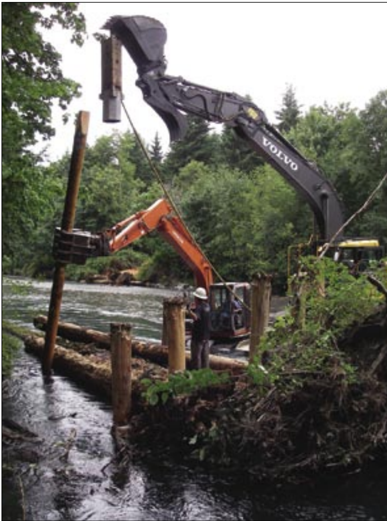
Construction of an engineered log jam on the Dosewallips River. Piles were driven to pin the structure into place. As one excavator holds the pile in place, a second excavator positions the pile driver above the timber.
