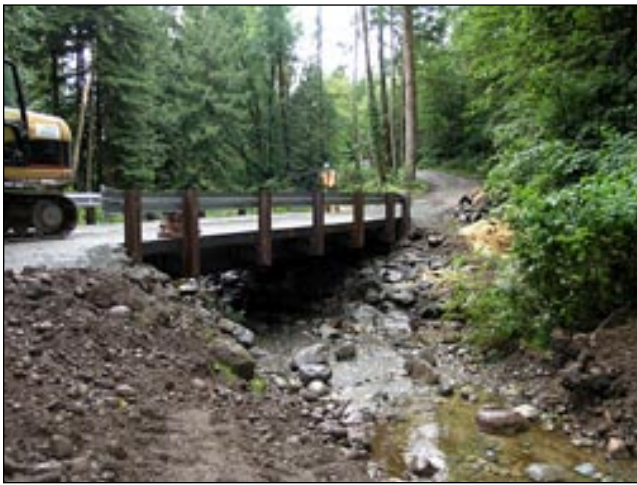
A new bridge improves fish passage and helps landowners in Weiss Creek.
