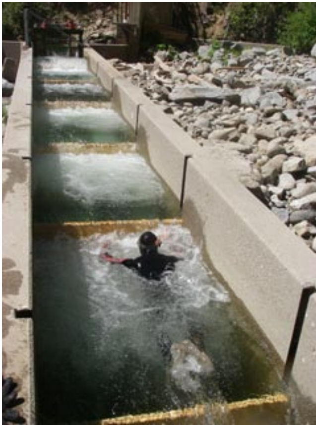
Renovated fish ladder at LNFH water intake dam. Structural improvements to facilitate fish passage were made by USFWS in July 2006.
