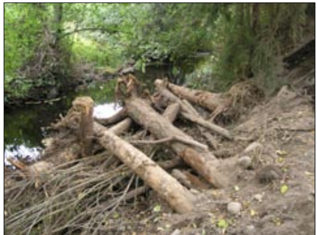
During summer 2006 WFC and the City of Olympia constructed four engineered logjams within Olympia's Black Lake Ditch. Photo by Jamie Glasgow.
