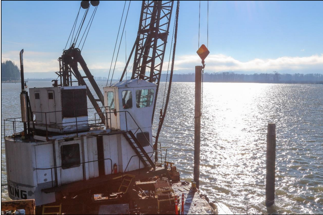
Figure A-2. Pile driving in December 2015. Photo by Kurt Beardslee (WFC 2018).
