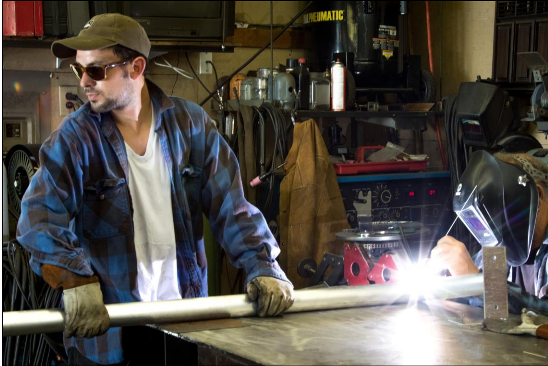
Figure D-4. Prefabricating components of the fish trap with STA-Weld (Redmond, WA).
