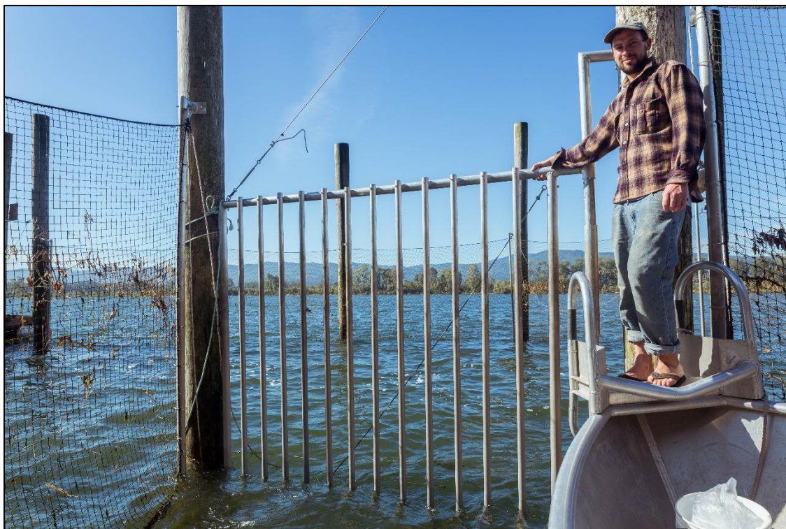
Figure V-2. Marine mammal gate deployed at the entrance to the heart of the trap to prevent entry of mammals and enable passage of fish.
