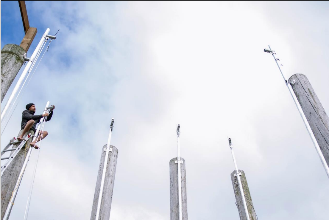
Figure D-8. Constructing the spiller compartment in August 2017.
