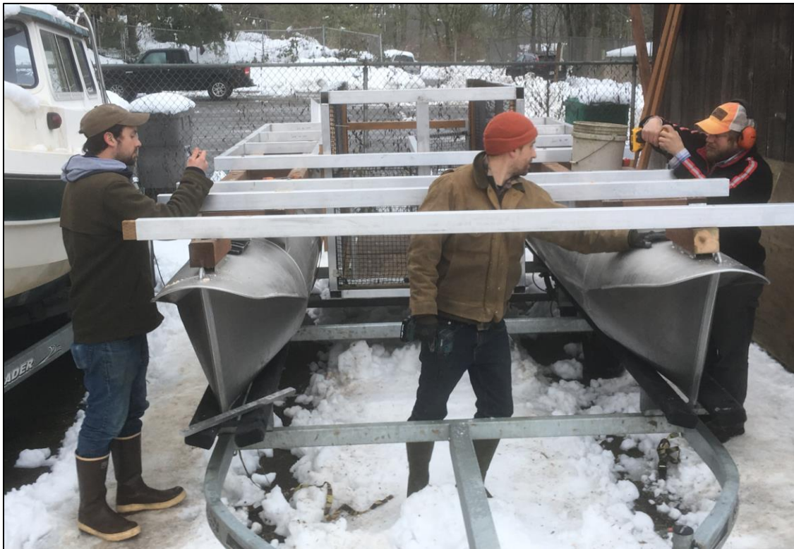
Figure D-24. Constructing the modified live well dock for passive capture in February 2019.
