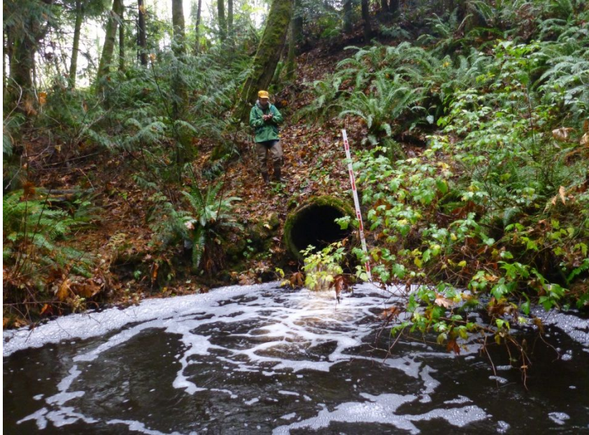
Miller Rd. NE Culvert outlet perched 1.3 ft into a large plunge pool.
