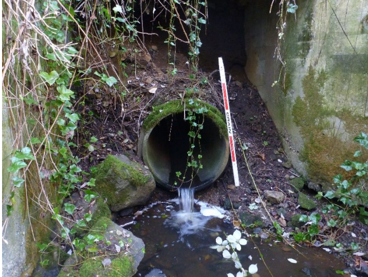
NE Country Club Rd. culvert outlet perched 1 ft with concrete retaining wall.
