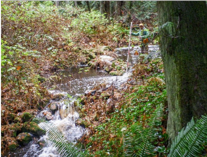
Two boulder weirs downstream from the Miller Rd. NE plunge pool.
