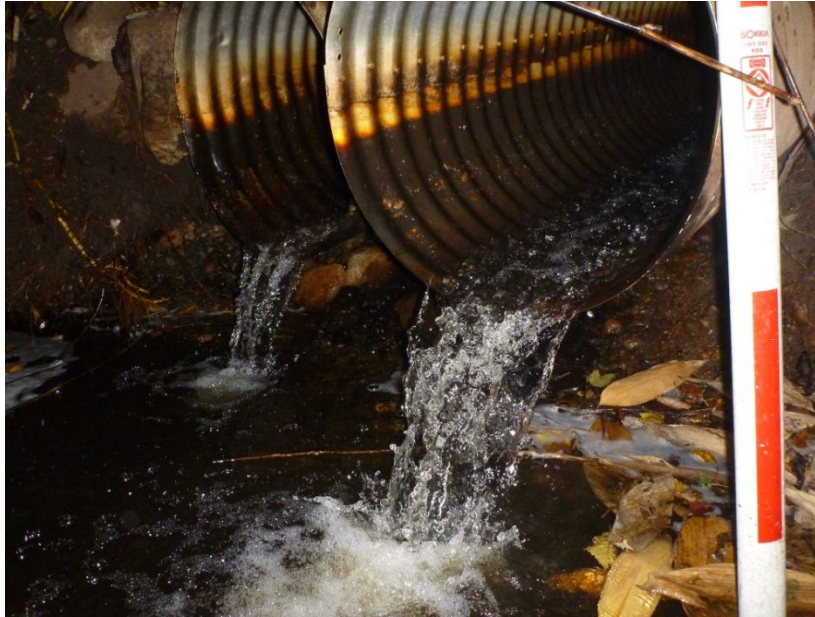
Outlet of the side by side culverts running under Miller Rd. NE. Perched 1 ft and undercut.
