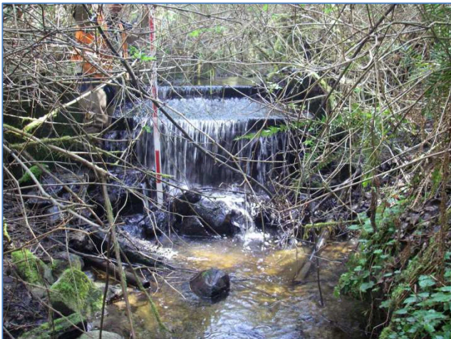
Looking upstream at the old dam structure outfall
