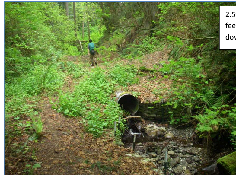
Reservoir where surface water is diverted into the hatchery. Remaining flows feed through 2.5' culvert and into the downstream channel.
