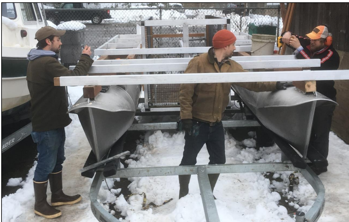
Figure A-1. Constructing the modified live well dock for passive capture in February 2019.
