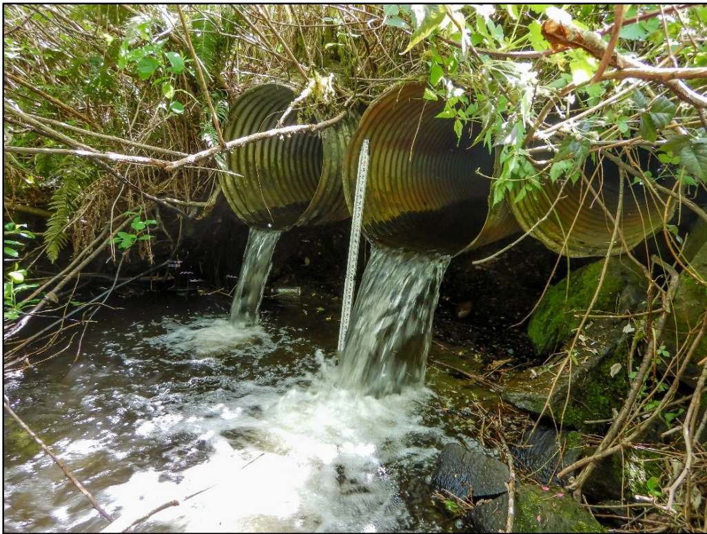
Figure A2. Barrier culvert outlets, perched approximately 2 ft. during the time of WFC survey.
