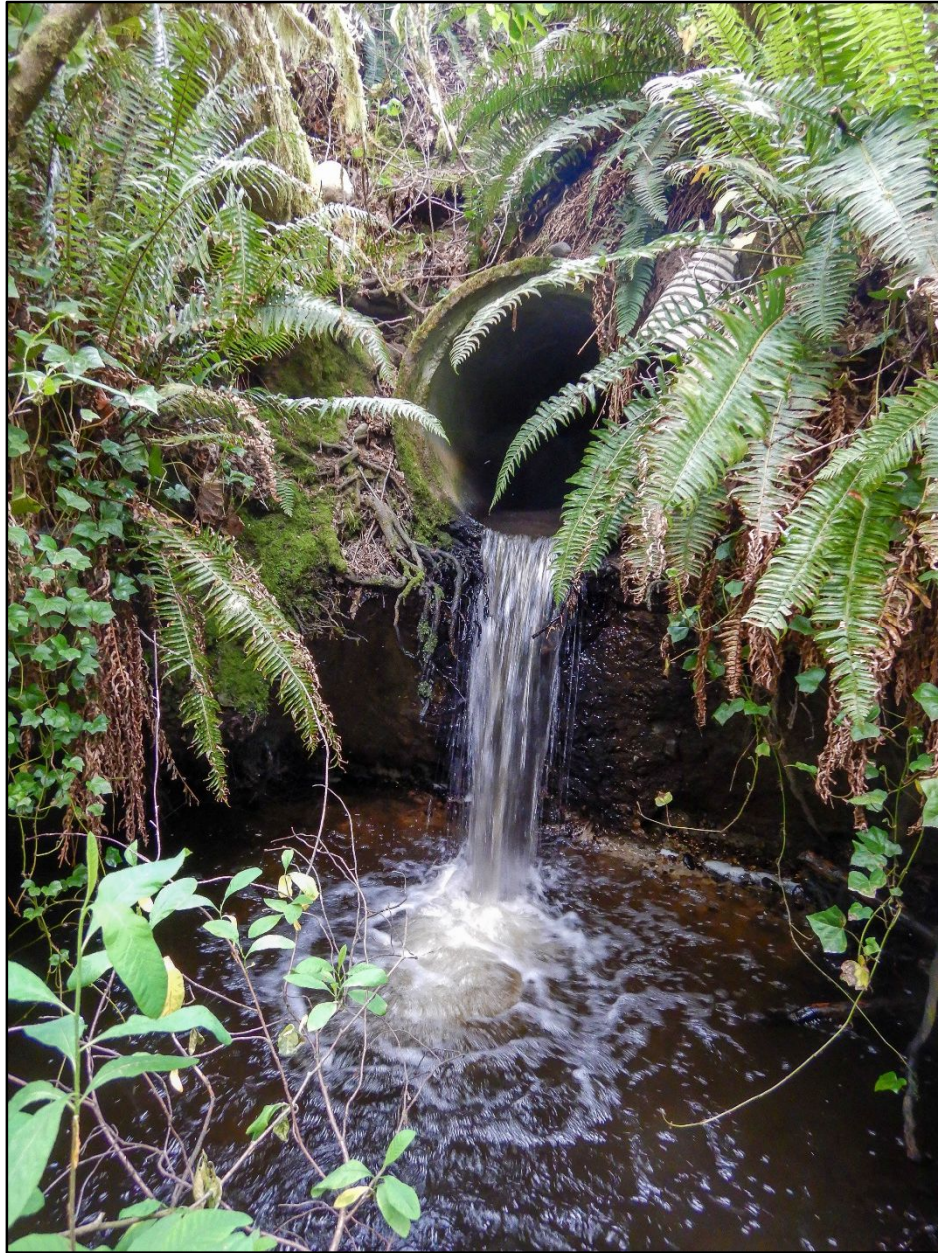
Figure C2. Barrier culvert outlet
