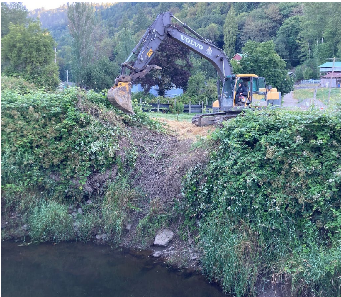
Exhibit 4-1: Photograph of Riprap Encountered in Test Pit TP-4b-22
